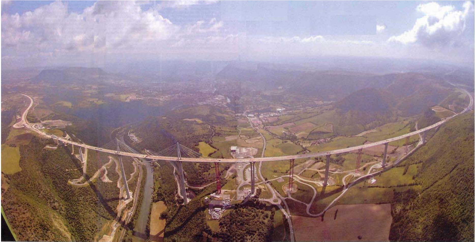
Millau Viaduct, France
